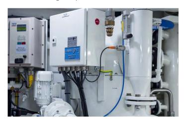
Waste water system: Hamann HL Plus 02 system, capacity 5,200 I / 1374 USG per day
