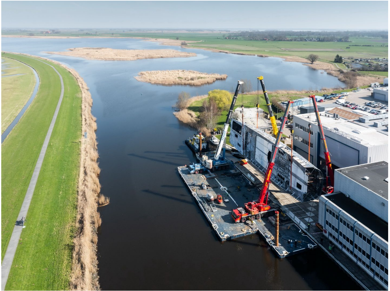
PRECISION LIFTING AND TURNING OPERATION AT THE VOLLENHOVE SHIPYARD
